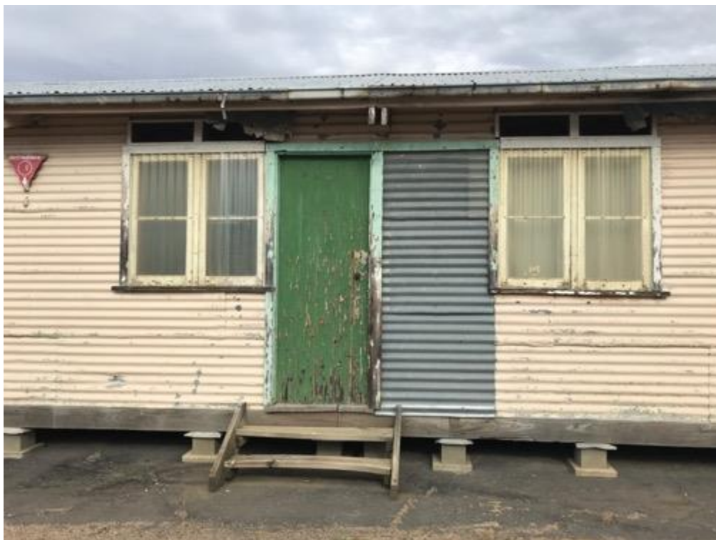
Detail of changes to door and window configuration – west elevation
