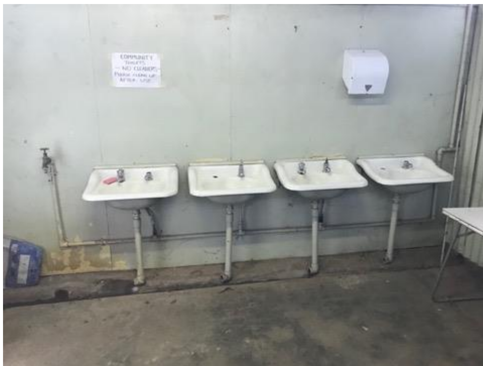
Wash basins – note the drainage into an open drain
