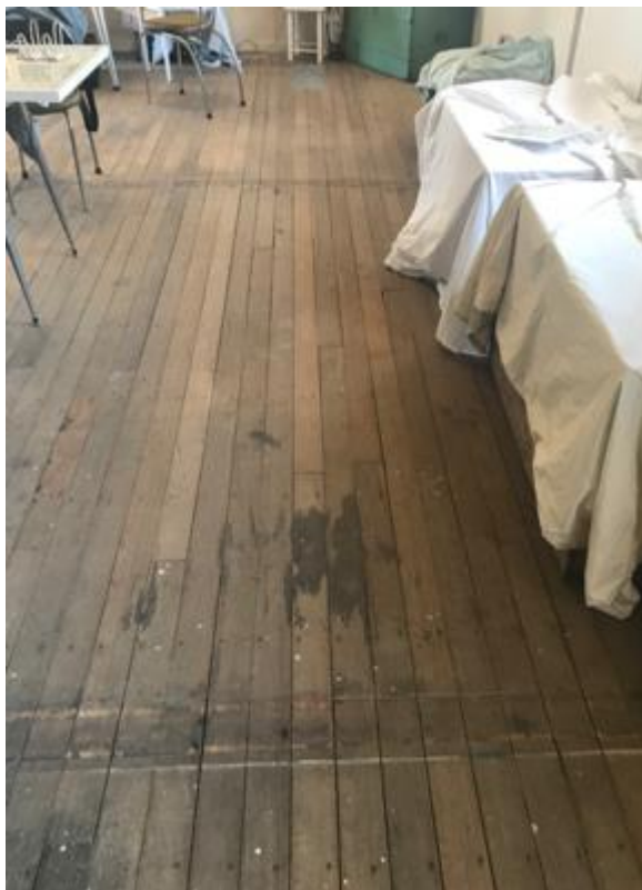
Evidence of the former walls - marks on floor
